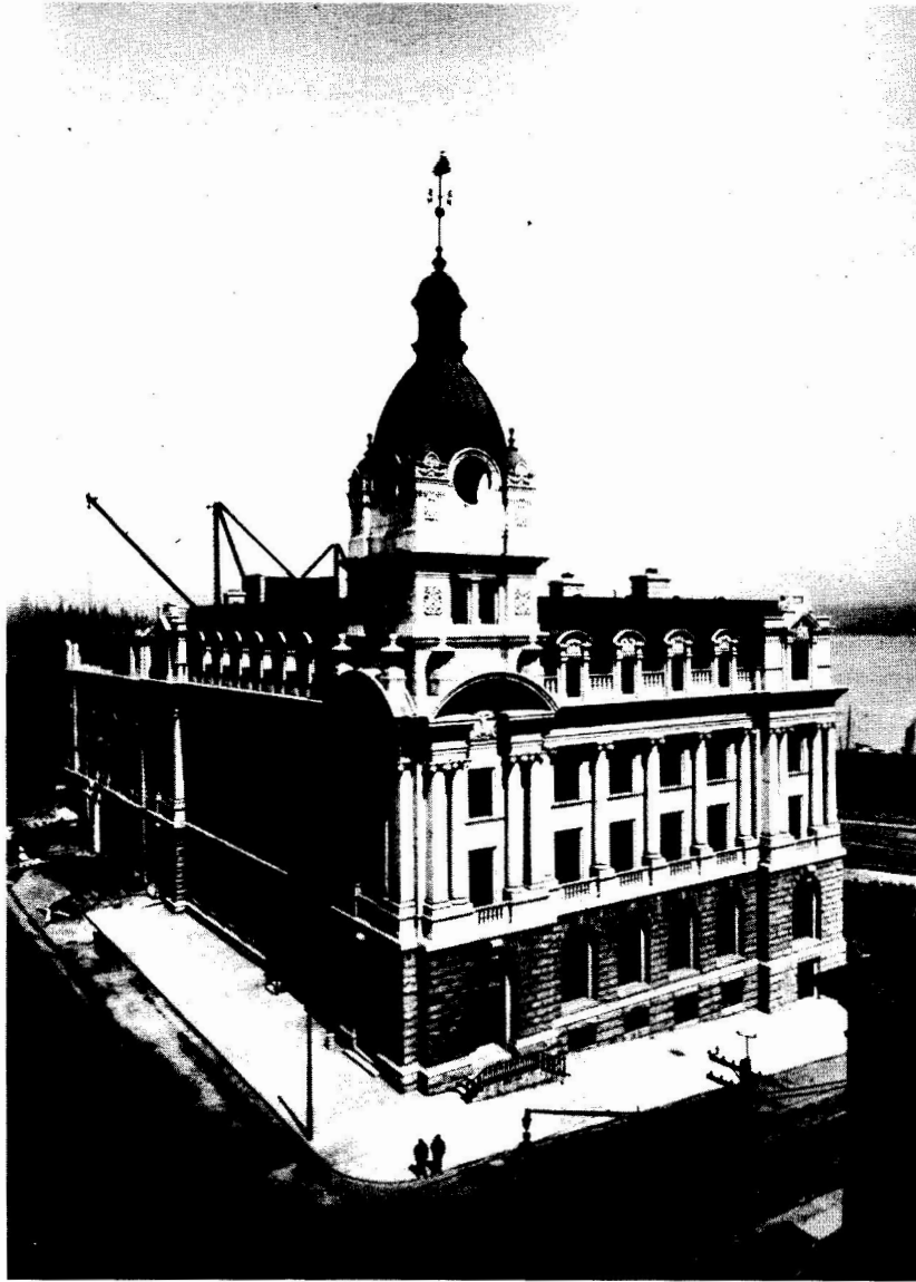
FIGURE I. POST OFFICE AND WINCH BUILDING UNDER CONSTRUCTION (CIRCA 1909)
