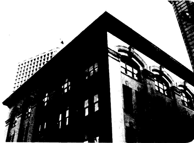
FIGURE 2. CORNICE ON ROOF OF CUSTOMS EXAMINING WAREHOUSE
